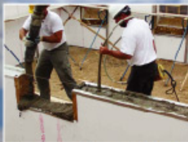
Concrete Consolidation
